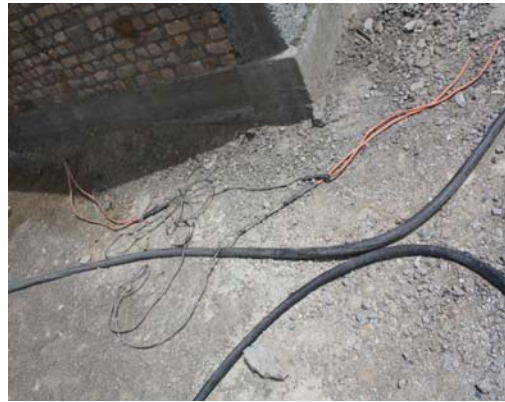
Figure 12. Spin Boldak: Taped splices (unlisted connectors) are exposed to the weather and cause an increased risk of electrocution during wet weather.
