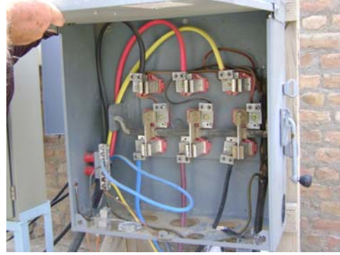
Figure 10. Spin Boldak: Connecting wires are undersized making them a fusible link, and there is no wire protection around the knock-outs at the bottom of the panel.
