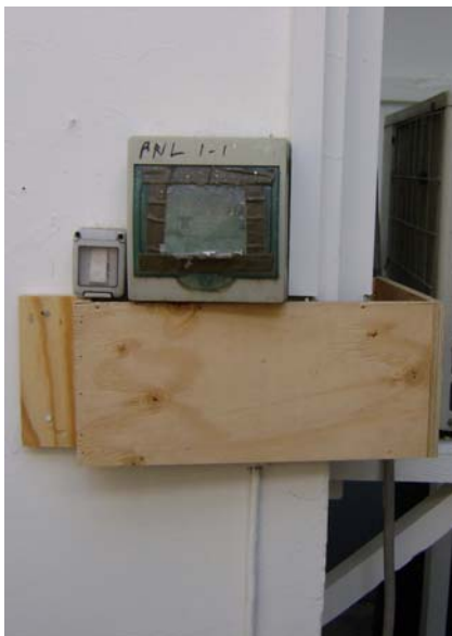
Figure 3. Temporary fix performed by contractor to protect personnel from coming into contact with exposed wires at Camp Eggers.
