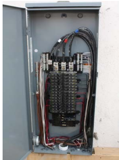
Figure 2. Color coding of wires by a contractor with tape to bring box into NEC compliance at FOB Altimur.
