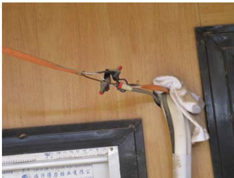
Figure 13. Spin Boldak: A sock used as an electrical insulator and an exposed splice is a fire hazard.
