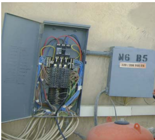
Figure 7. Camp Brown: The undersized wire will melt before the breaker trips causing a fire and blast hazard. Panel on the left has no dead front causing a blast hazard.
