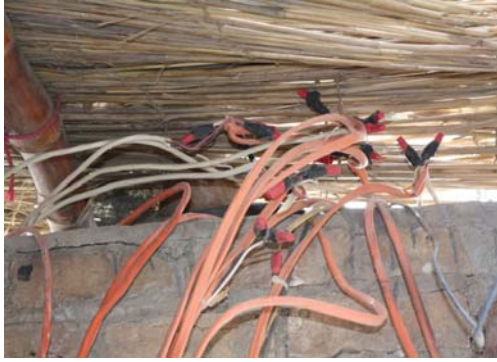
Figure 9. Spin Boldak: Exposed splices directly below an exposed straw roof create a fire hazard, and the splices are not weather-protected.
