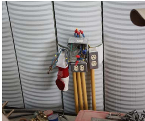
Figure 6. Camp Brown: Electrical re-wiring, to correct work performed by an untrained worker, was performed by a Seabee to prevent injury or property damage.
